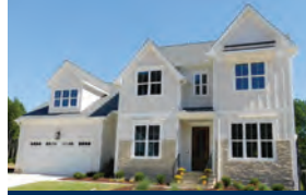
UPRIGHT BUILDERS Lot 163: 84 Autumn Gate St.
